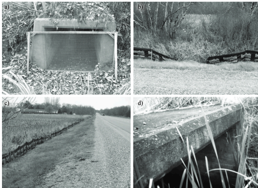
Grate treatment (a), fence treatment (b, c), and control (d) sites (Cunningham et al. 2024).
